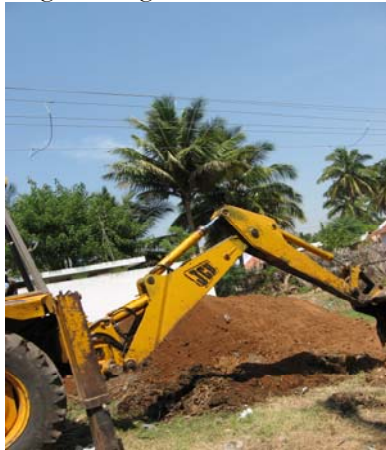
Compost pit ready
