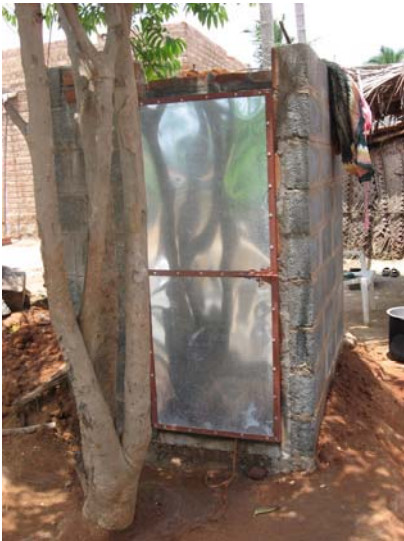
One IHHL being constructed
