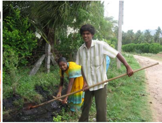
The ditches being cleaned
