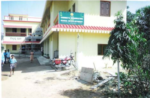
CORD Building at a Glance
